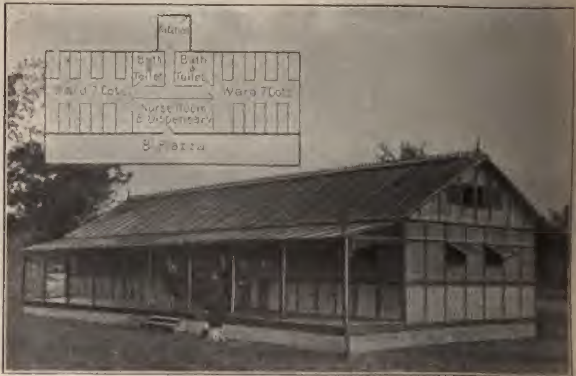
FIG. 202.— Portable hospital pavilion, system Ducker.
